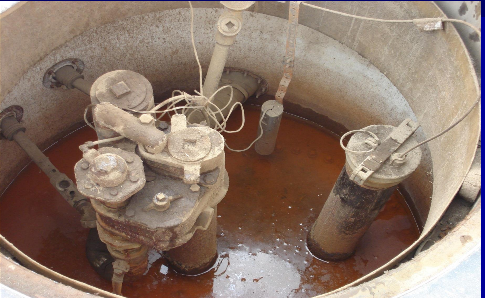
Liquid in sump
